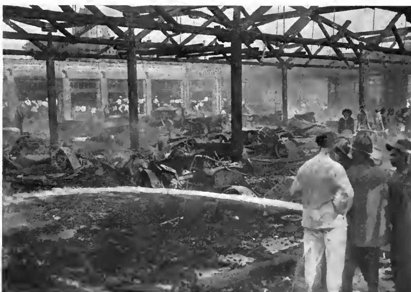
FIG. 2. A RECENT UNSPRINKLERED GARAGE FIRE IN YAKIMA, WASHINGTON
